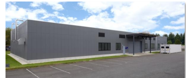
Tochigi xEV Battery Safety Test & Certification Center Utsunomiya City, Tochigi Prefecture
