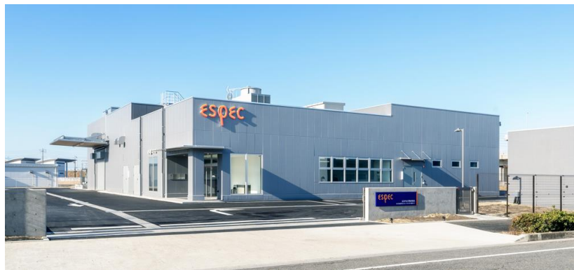
Aichi xEV Battery Safety Test & Certification Center (Tokoname, Aichi Prefecture)
