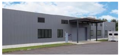
Battery Safety Testing Center
