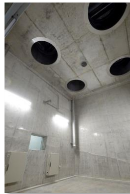
No. 2 Safety Test Room
