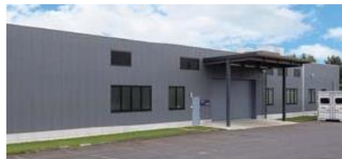
Battery Safety Testing Center
