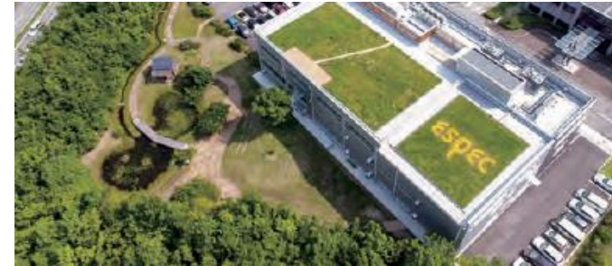
Rooftop green space using only native species
