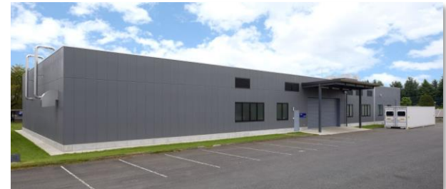
Battery Safety Testing Center
