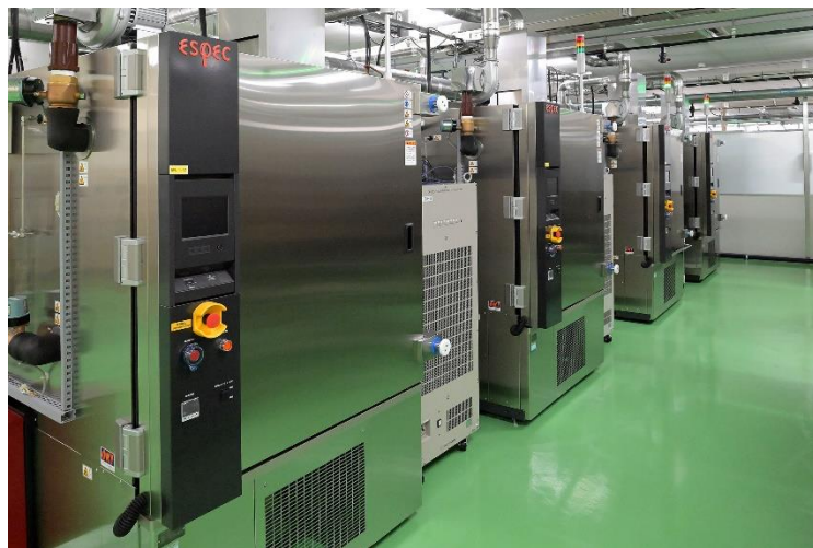
SoftBank Next-generation Battery Lab Inside the ESPEC Battery Safety Testing Center
