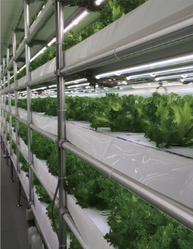
This plant factory can produce vegetable year-round by using artificial light source such as LEDs, and it can be also customized to each productions scale according to your requirement.
