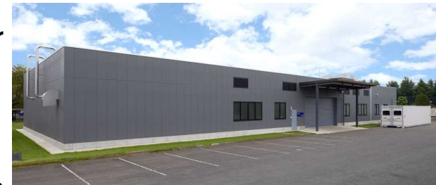
Battery Safety Certification Center (in Utsunomiya Technocomplex)
