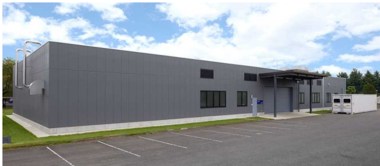
Battery Safety Certification Center (in Utsunomiya Technocomplex )
