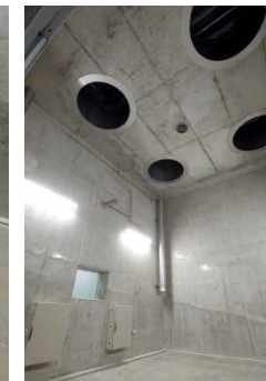
No. 2 Safety Test Room
