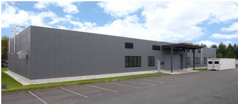
Battery Safety Certification Center (in Utsunomiya Technocomplex )
