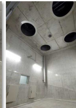
No. 2 Safety Test Room
