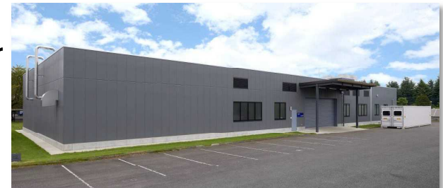
Battery Safety Certification Center (in Utsunomiya Technocomplex)
