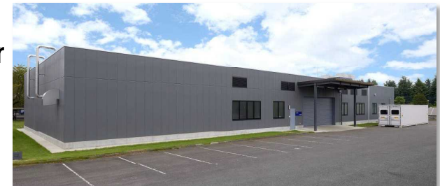
Battery Safety Certification Center (in Utsunomiya Technocomplex)
