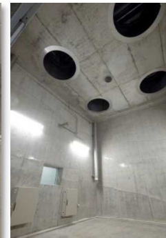
No. 2 Safety Test Room
