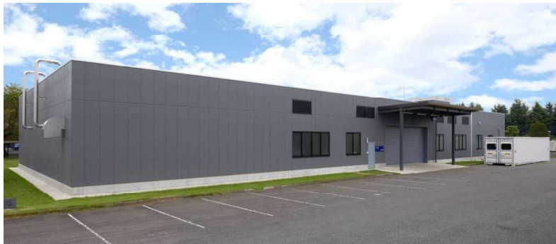
Battery Safety Certification Center (in Utsunomiya Technocomplex )
