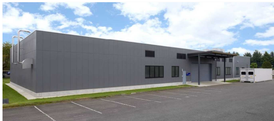
Battery Safety Certification Center (in Utsunomiya Technocomplex )
