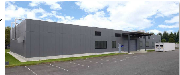
Battery Safety Certification Center (in Utsunomiya Technocomplex)
