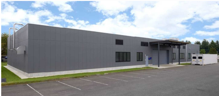
Battery Safety Certification Center (in Utsunomiya Technocomplex )
