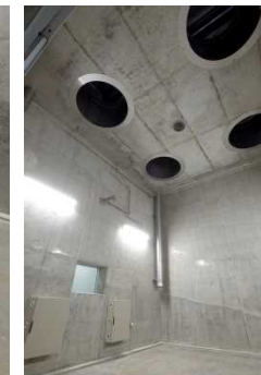
No. 2 Safety Test Room
