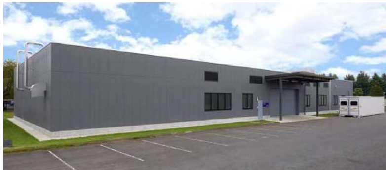
Battery Safety Certification Center (in Utsunomiya Technocomplex )
