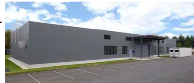
Battery Safety Certification Center (in Utsunomiya Technocomplex)
