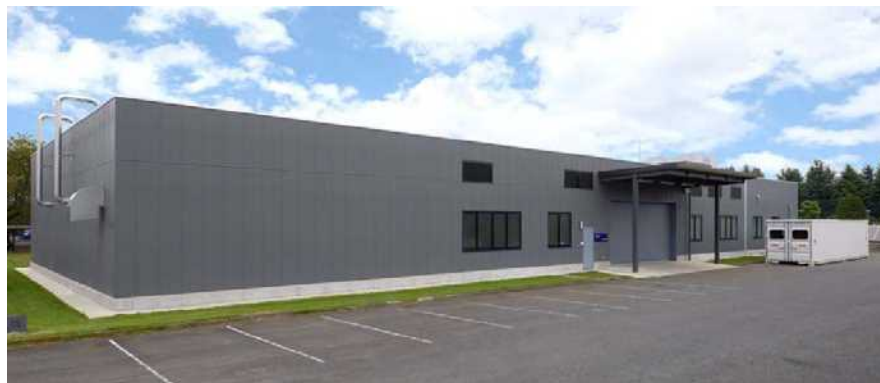
Battery Safety Certification Center (in Utsunomiya Technocomplex )
