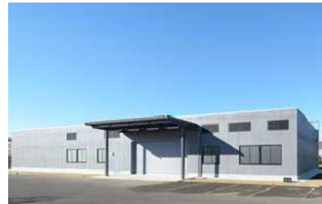
Energy Device Environmental Test Center
